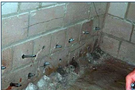
Place the injection packer into the hole. Tighten by using a ratchet and socket or an open-end wrench by turning clockwise as tightly as possible.
