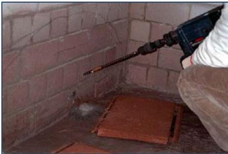
Clean the surface of the leak area. These will help technician to identify the exact location and width of the crack prior injection. Sometime the concrete surface hidden under the deposit of dirt and dust for long time. You must remove and clean the surface to see the crack line.
