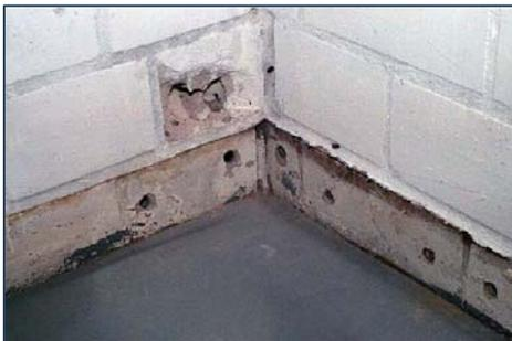
Install the entry ports (Injection packers). The size and depth of packer depend on the width of walls or floors.
