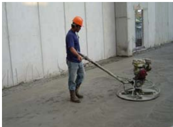
Apply by trowel
